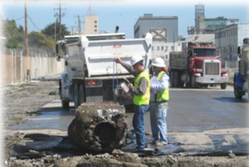
Soil and Sewer Line Removal
