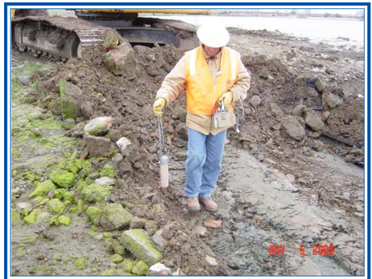
Technician Performing Radiological Scan While Excavating at Parcel E
