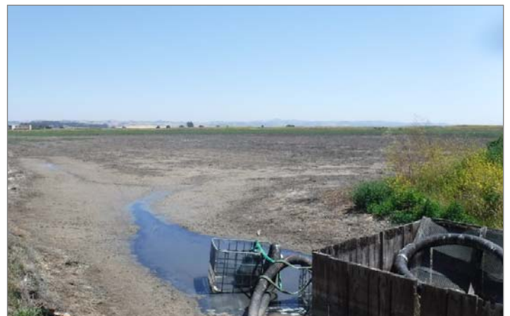
UXO 3—Dredge Pond 3E Dewatering June 8, 2018
