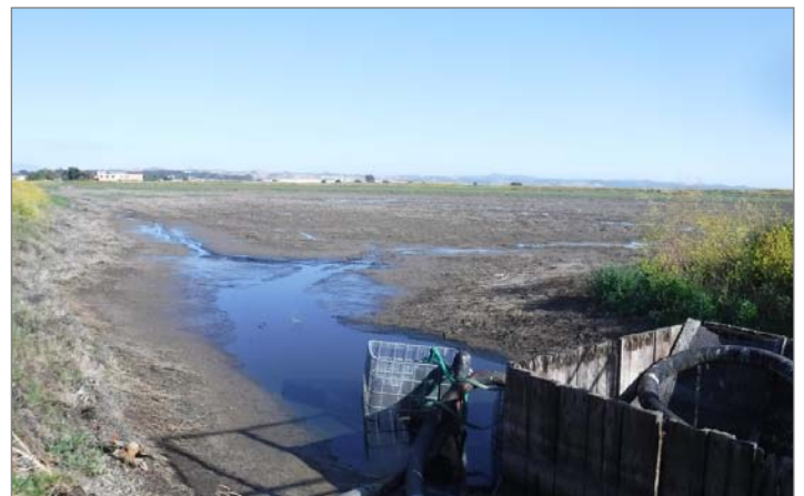
UXO 3—Dredge Pond 3E Dewatering June 5, 2018
