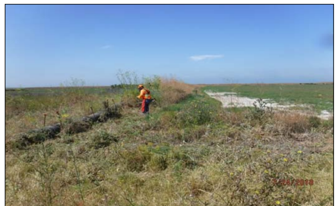
Vegetation clearance at UXO 3—Dredge Pond 3E (hand-held equipment) - July 24, 2018
