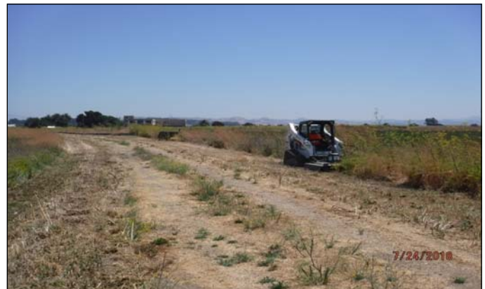
Vegetation clearance at UXO 3—Dredge Pond 3E (skid steer equipment) - July 24, 2018
