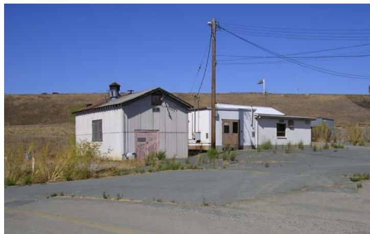
Site 27 Boiler House (Bldg IA-36) and Chemical and Materials Testing Laboratory (Bldg IA-20)
