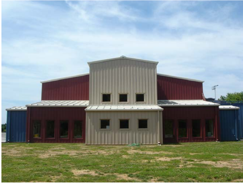
Children's Theatre of Annapolis Building – Southwest View
