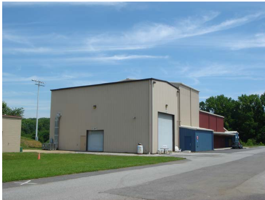
Children's Theatre of Annapolis Building and Building 217 – North View
